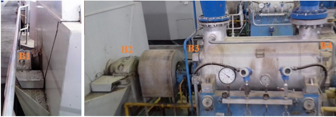
Figure 1. Pump Bearing Positions.
